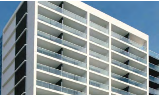
White concrete frame
